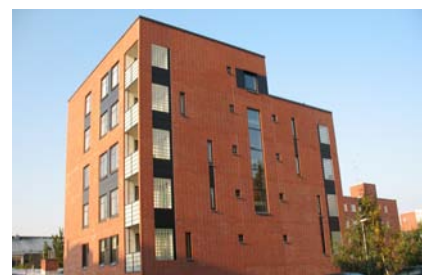
Exterior wall constructed of concrete tiles giving the appearance of brick
